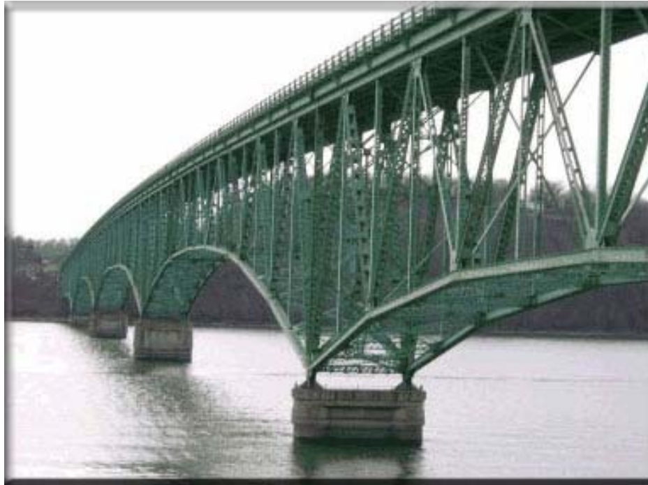
Hurricane Deck Bridge located at the Lake of the Ozarks
